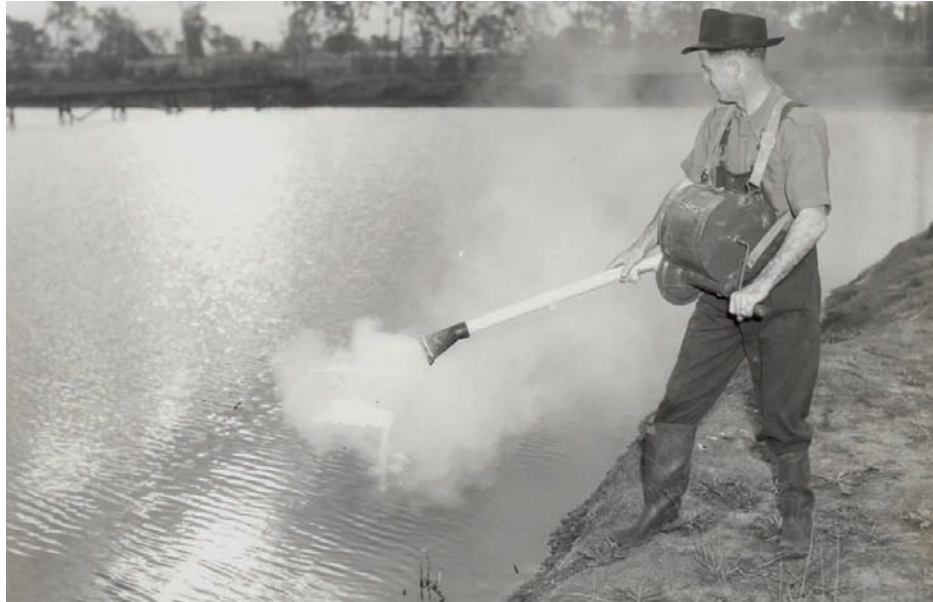
Fig 3. A duster used for applying insecticides by Vector Services. Date unknown.
